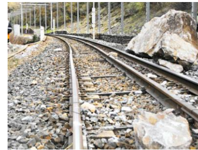
Obstacles on the rail
